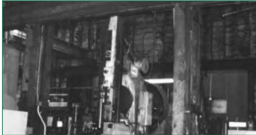
The old hay barn's high ceilings allow for 10-ton cranes over all the machines
